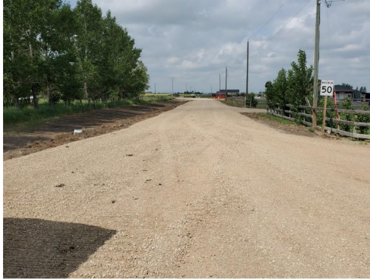
Figure 2. Twp Rd 6-1A East of Rng Rd 21-2
