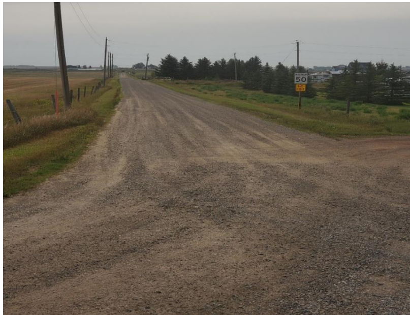
Figure 5. Twp Rd 6-3A East of Raymond Shop
